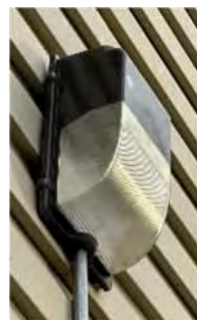
Figure 23 – LED Mini Wall Pack (LMWP)
