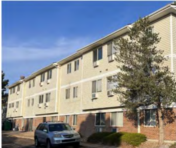
Figure 8 - Partial South Facade
