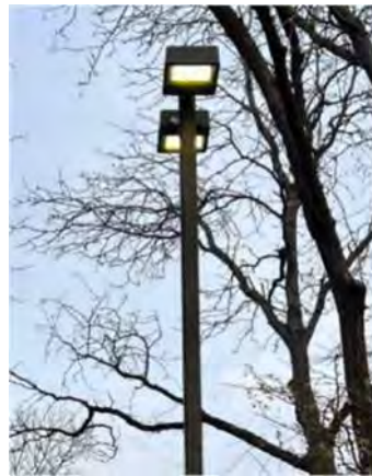
Figure 21 – LED Parking Lot Light (LPL)
