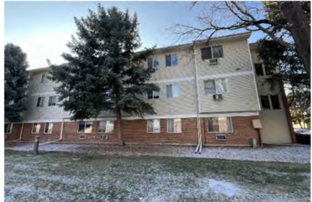
Figure 5 - Partial North Facade
