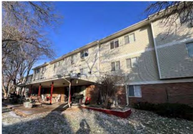
Figure 4 - Partial South Facade
