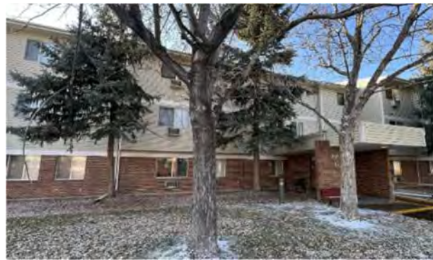
Figure 9 - Partial North Facade
