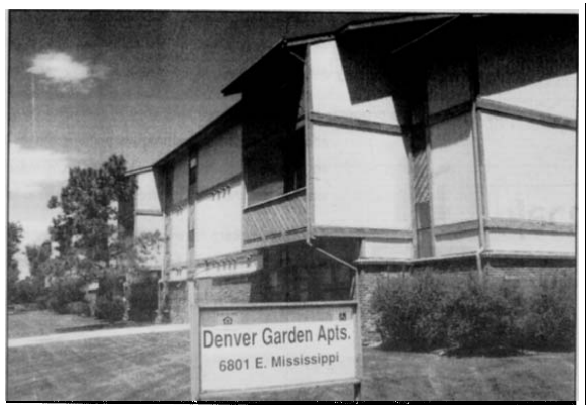
Community Housing Concepts Inc. is CHFA's first Tax Credit Assistance Program recipient. The funds support the Denver-based nonprofit's plans to preserve the affordability and renovation of the 100-unit Denver Gardens Apartments.
